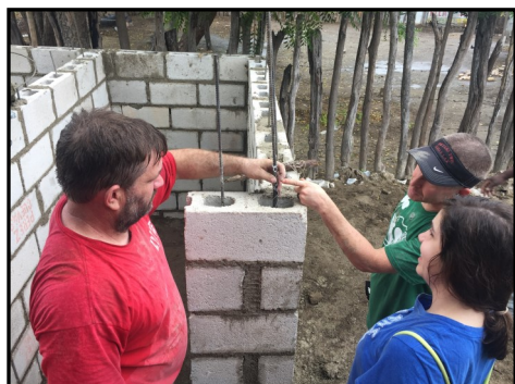
A lesson on joining rebar.
