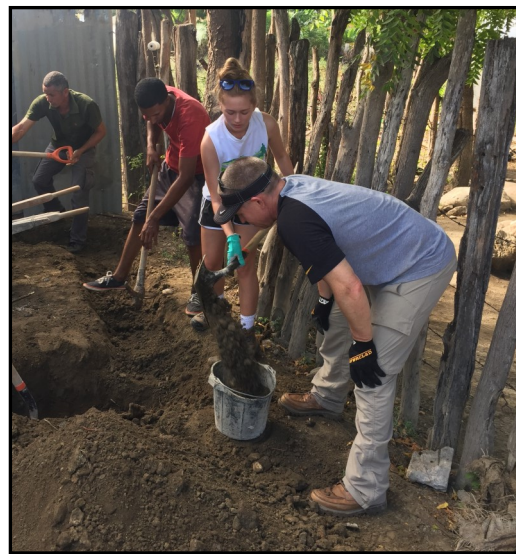
Digging the footers for the bathrooms in Batey 2.
